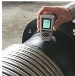
Paint Thickness Inspection
